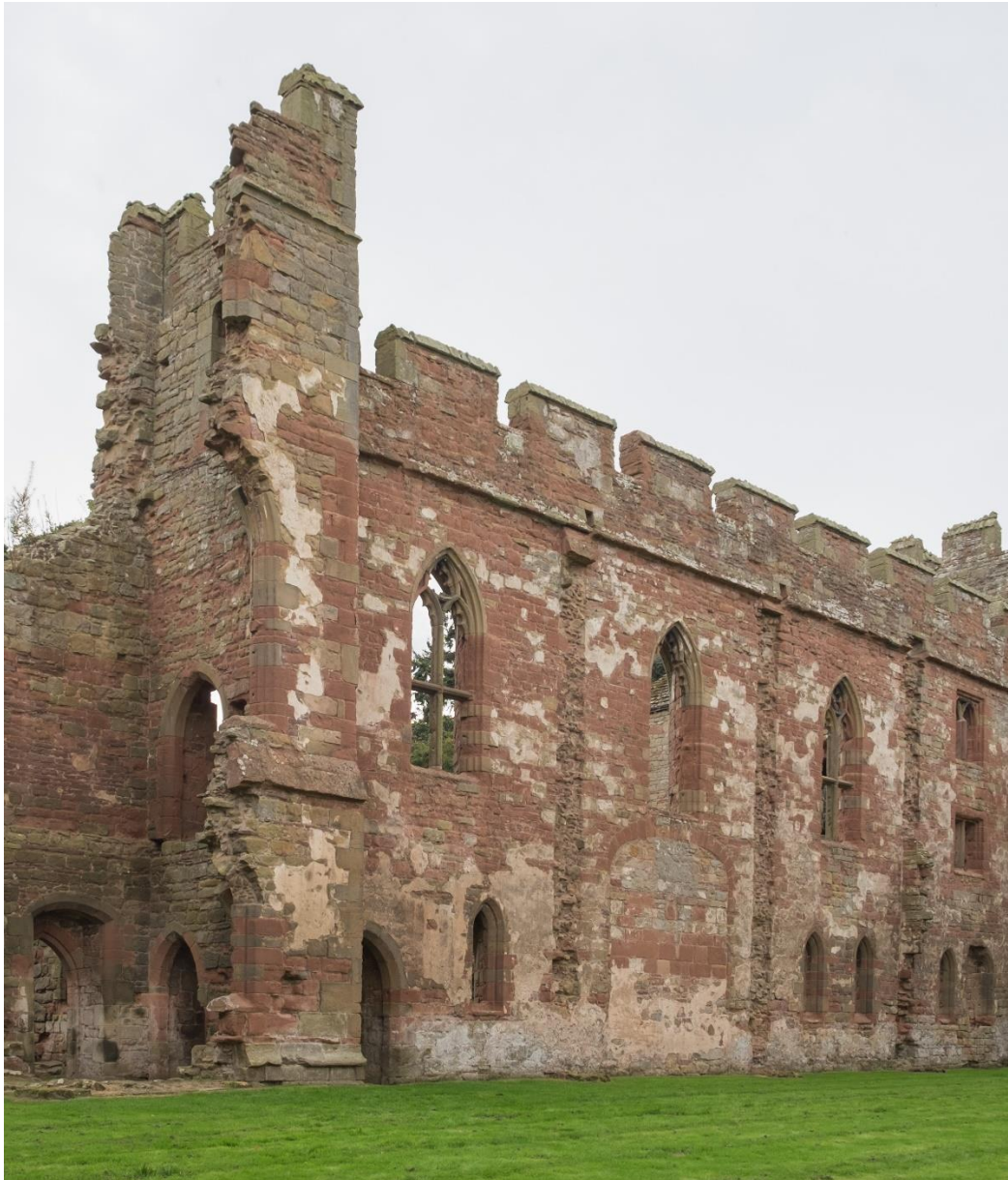
Image 3: Evidence of lime render/whitewash on exterior of Acton Burnell Castle- 1280s
