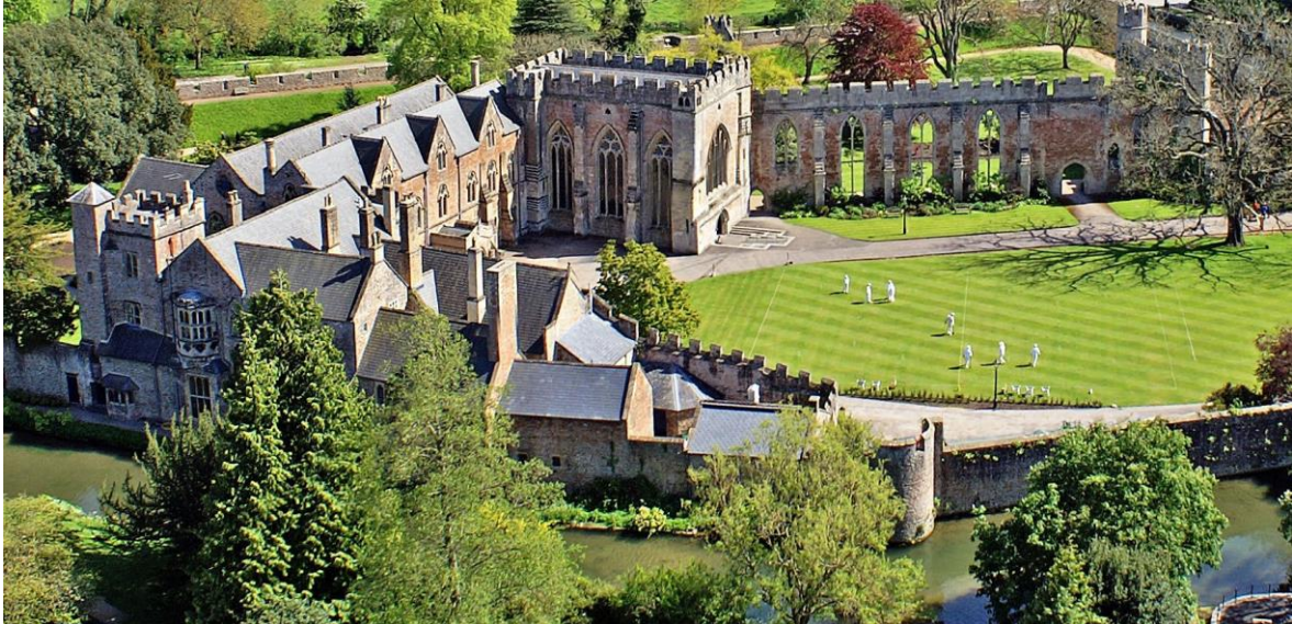
Overview of The Bishop's Palace, Chapel and Moat.
